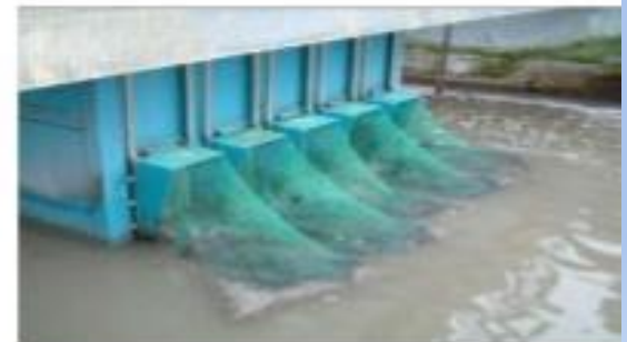
Coarse screener for large floating garbage and twigs.
