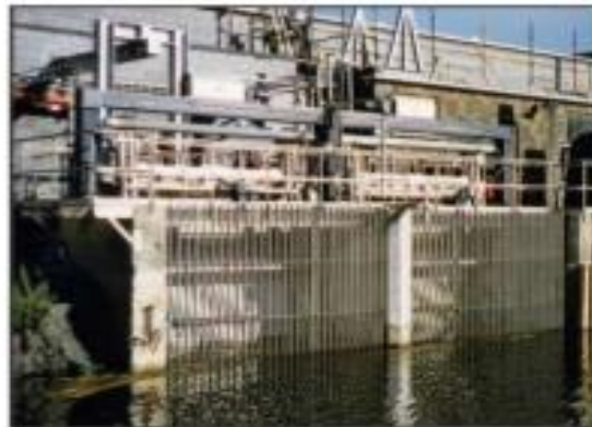
Coarse screener for large floating garbage and twigs.
