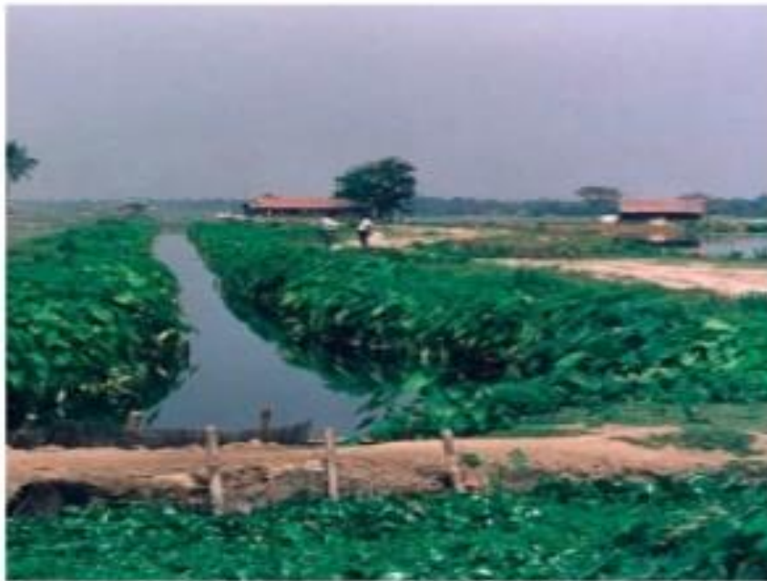
Open channel through which sewage is flown to the pond.
