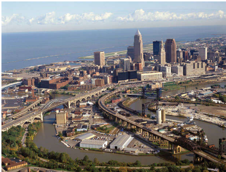
FIGURE 19.10 The Cuyahoga River (lower left) flows toward Cleveland, Ohio, and the Erie Canal (lower right) is in the Cuyahoga National Park. The skyline is that of industrial Cleveland.
