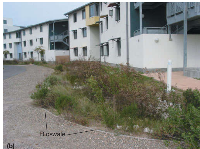
FIGURE 19.12 Bioswales collect runoff from Manzaneta Village Dormitory Complex at the University of California, Santa Barbara. (a) Plants in bioswales (b) help filter water and remove nutrients, reducing cultural eutrophication.
