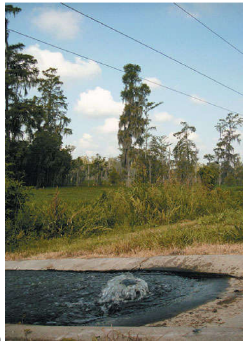
FIGURE 19.18 (a) Wetland Pointe au Chene Swamp, three miles south of Thibodaux, Louisiana, receives wastewater; (b) one of the outfall pipes delivering wastewater; and (c) ecologists doing field work at the Pointe au Chene Swamp to evaluate the wetland.
