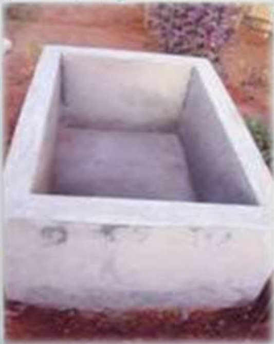
1. Tank for mass multiplication of AM
