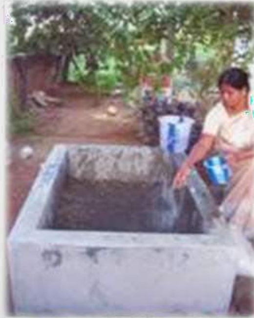
2. Sprinkling of water in tank with vermiculite
